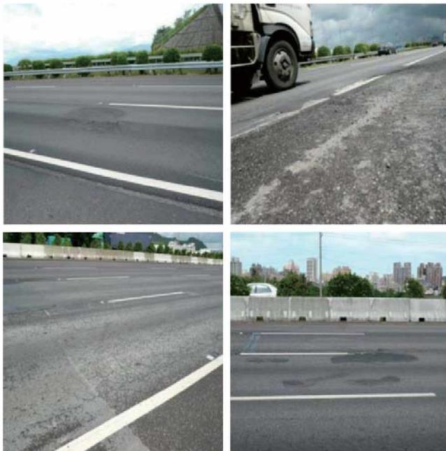
Fig. 7. Different types of potholes. The upper-left one is pavement rutting; the upper-right one is aggregate losses; the lower-left one is fatigue crack, and the lower-right one is pothole repair. Photo courtesy of [26].
